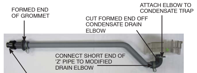
DRAIN ELBOW "Z" DISCHARGE PIPE FOR LEFT SIDE DRAIN IS ROUTED BEHIND INDUCER
